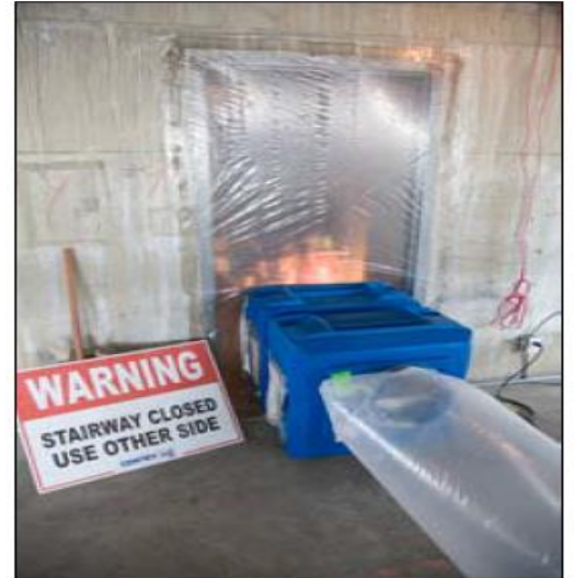
Poly enclosure with HEPA "negative air" unit
